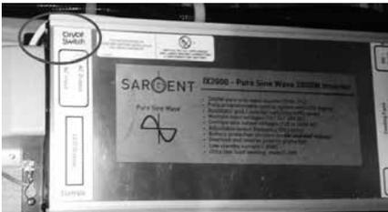
If no other source is available, the inverter will supply 230v power to the sockets in the appropriate list above, converting 12v power from the leisure batteries into 230v power at the sockets.
