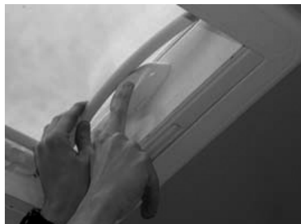
To open depress the button (Fig. A).
