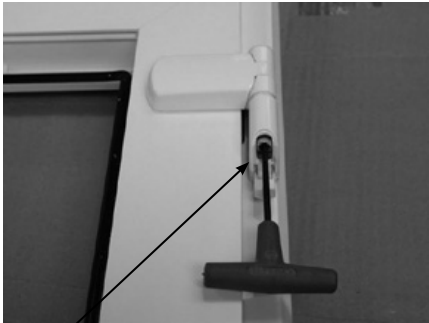
This bolt is used to adjust height and compression.
