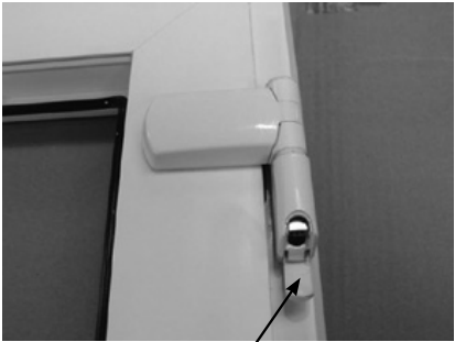
To adjust the door vent compression and height within the frame, unclip the cap as shown.
