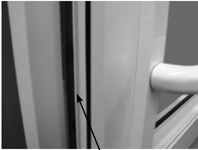
Adjusting the hinge as shown will correct this clearance.
